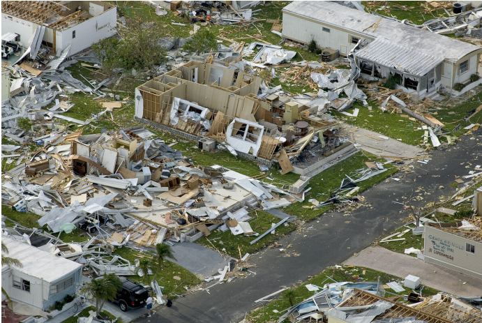
Damage Done by Hurricane Katrina
